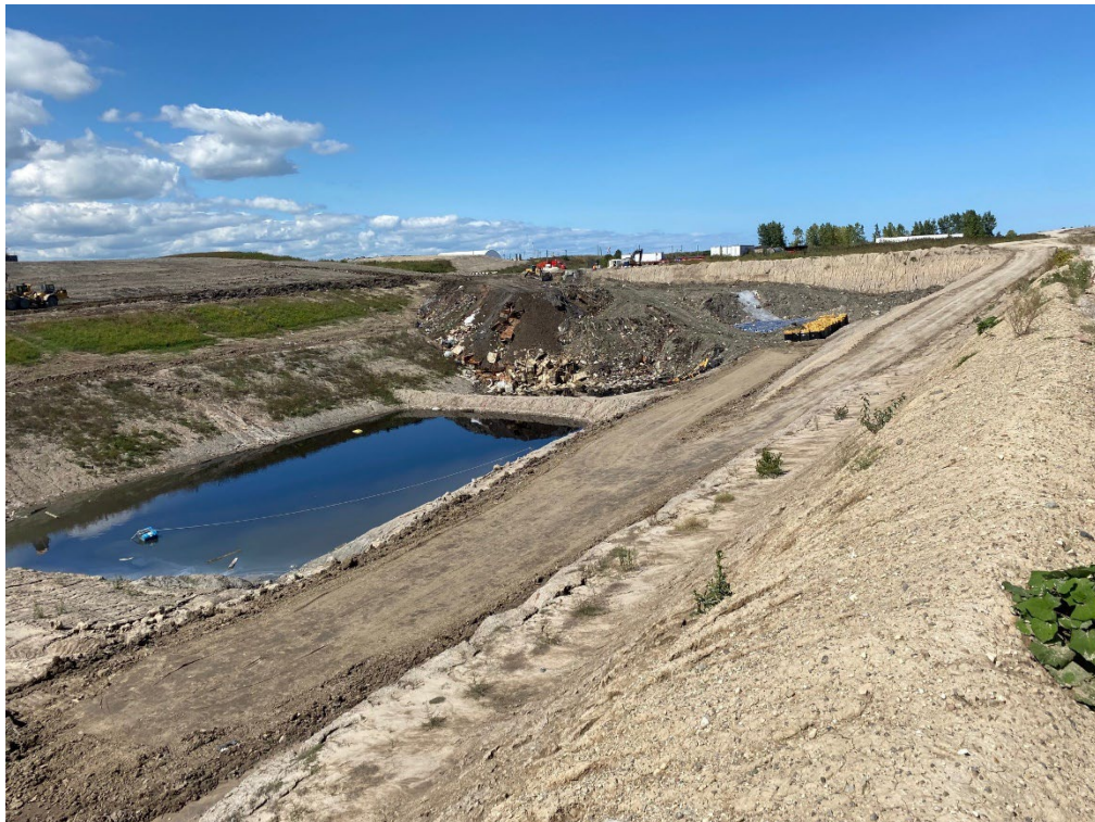
Photo 12- Cell 20-1, looking north, September 14, 2023..
