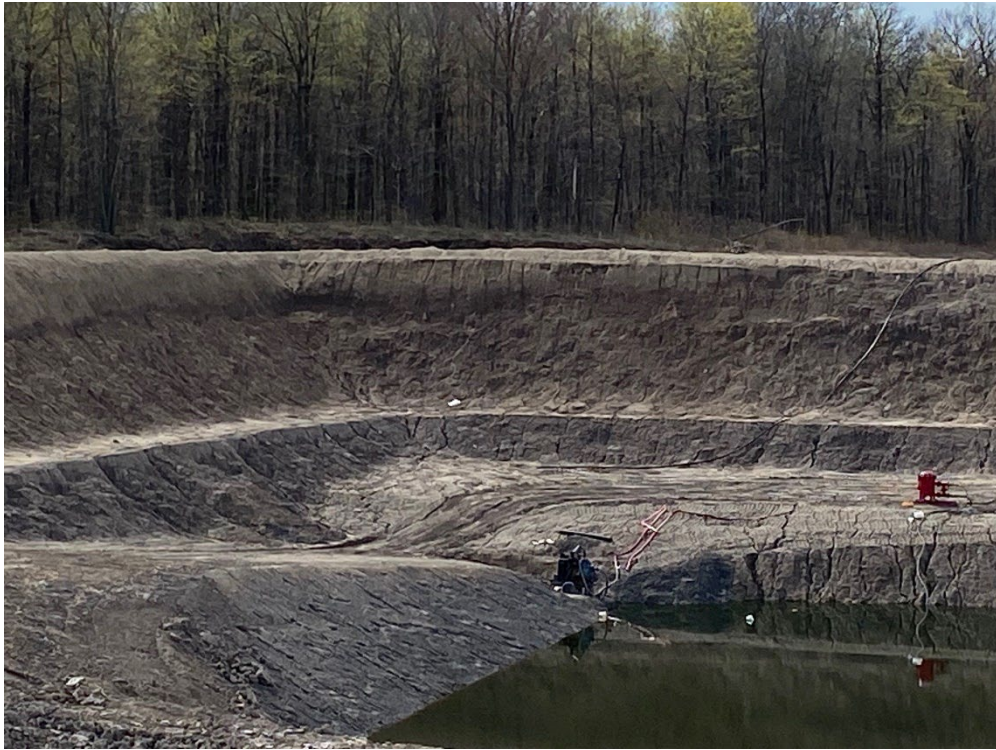
Photo 3- Cell 20-1 Southeast corner, April 19, 2023.
