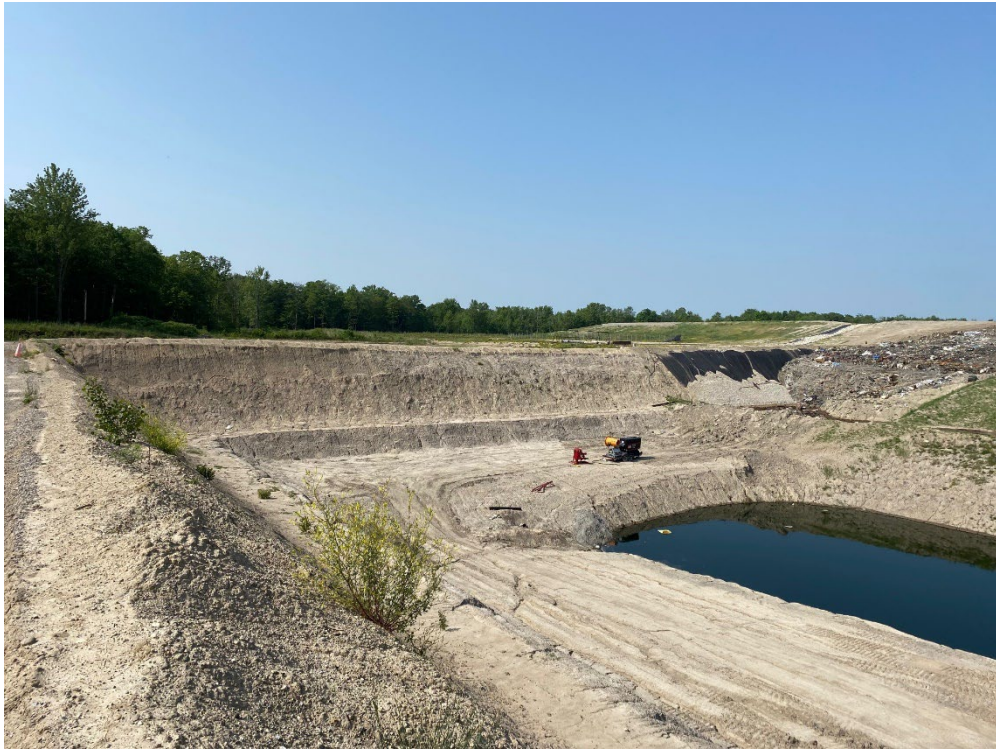
Photo 7- Cell 20-1, South side wall, June 21, 2023.
