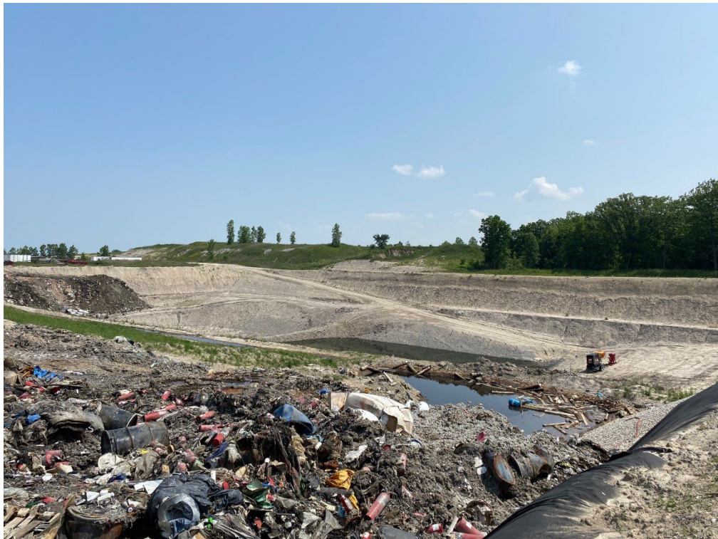
Photo 10- Cell 20-1, East and North side wall, looking east, June 21, 2023.
