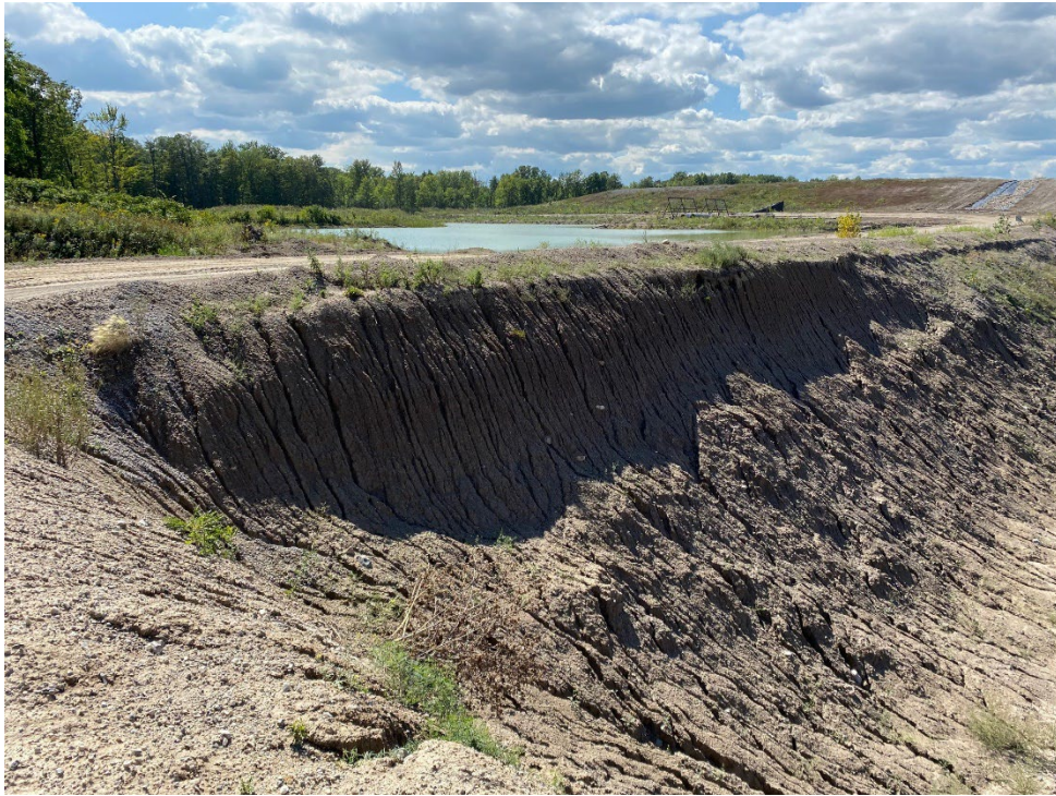
Photo 13- Cell 20-1, southeast corner, September 14, 2023.
