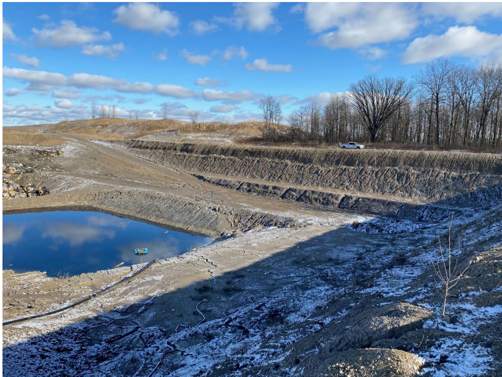
Photo 18- Cell 20-1, East side wall, December 19, 2023.
