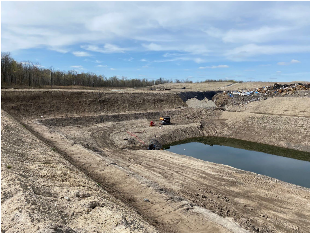
Photo 5- South side wall, April 19, 2023.
