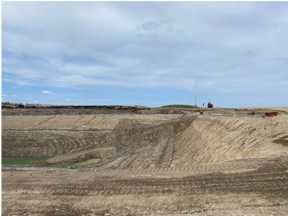
Photo 4- North side wall, April 19, 2023.
