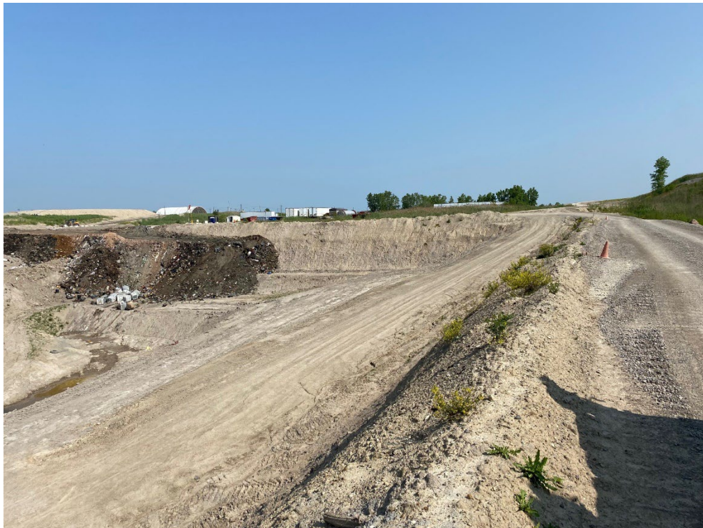
Photo 8- North side wall, start of waste placement, June 21, 2023.
