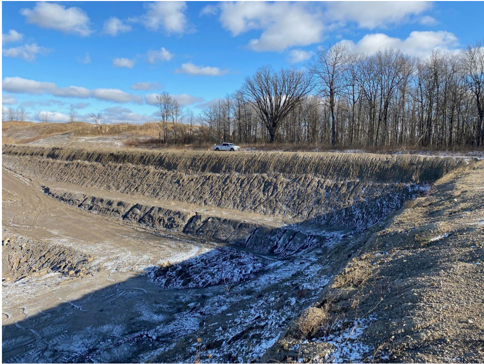
Photo 17- Cell 20-1 East side wall, December 19, 2023.
