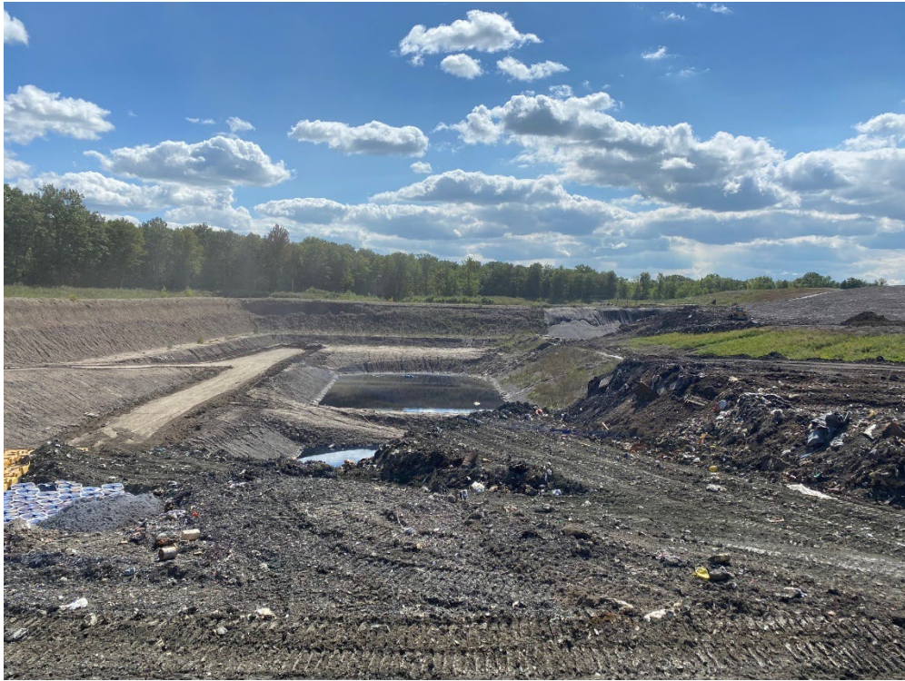
Photo 11- Cell 20-1, looking south. September 14, 2023.
