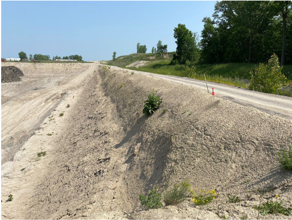
Photo 9- Cell 20-1, East side wall, looking north, June 21, 2023.
