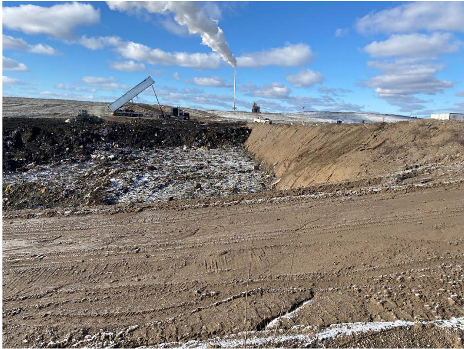
Photo 15- Cell 20-1, North side wall, looking west, December 19, 2023.
